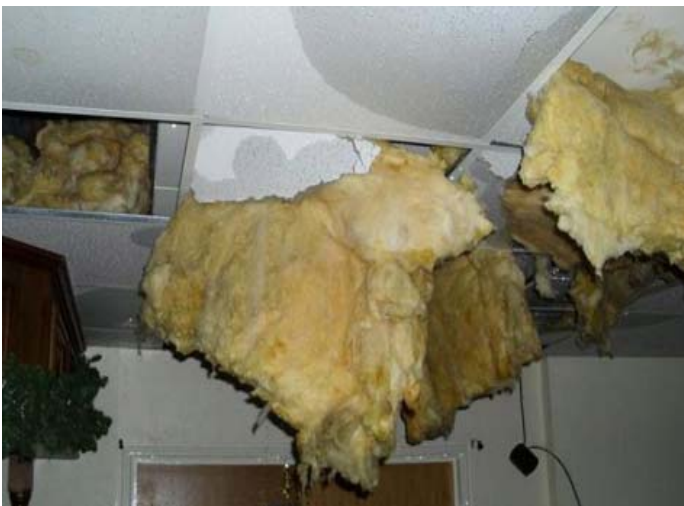
Ceiling panels brought down by a burst pipe in the roof
