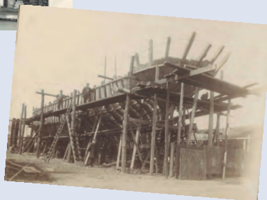
Photograph of a boat in construction at Hewett's Dock. NRO, Y/TC 69/23
