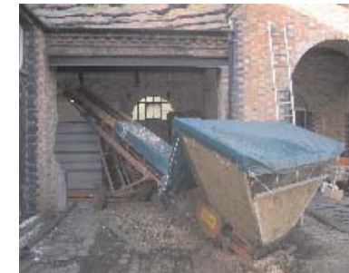
woodchip hopper and converted potato elevator
