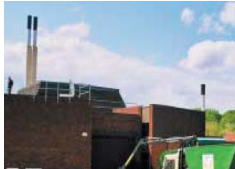
Wood-fuel flues can be small. In the above picture, the small chimney in the distance services the woodfuelled appliance and the large chimneys in the foreground belongs to the fossil-fuelled system that it replaced.
