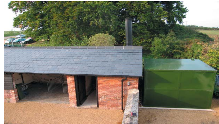
Boiler Room and woodchip storage hopper
